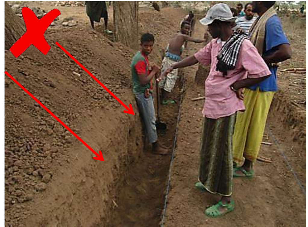
አፈሩ ተመልሶ ወደ ጉድጓዱ እንዳይገባ ጠርዙ ላይ አለማስቀመጥ:: Never place the soil close to the excavation site. It will fall back in.
