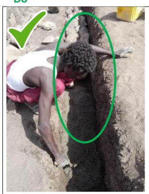
Stones are put together with the cementat the same time.
