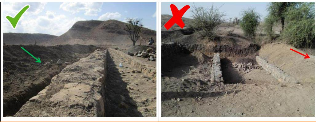
Soil is placed at the upper side of the weir.
