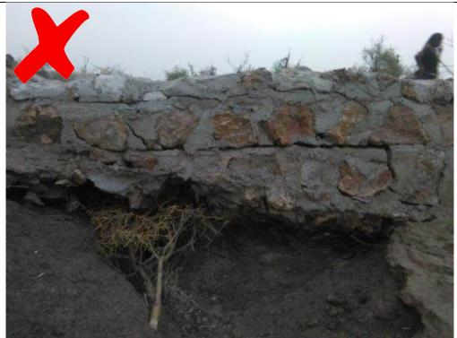
Never do shallow excavation. The water will wash the soil away below.
