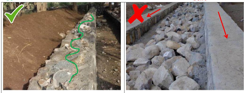
Build rough surface for the weir. The speed of water slows down.
