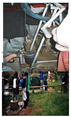
Mark the top end of the riser main on the side on which the catcher pipe of the guide box is to be situated. This is needed to ensure that the guide box (at the bottom) and the pump (on top) are properly aligned after installation. If this is not done carefully the rope and pistons might become entangled around the riser main and get stuck.
