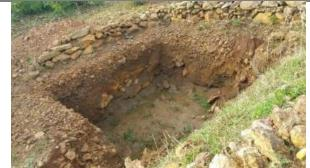
Fig. 2. Function of percolation ponds in the capturing of silts. See the flood mark from the side of the inner pond and feel the water that has soacked instead of being lost as runoff.
