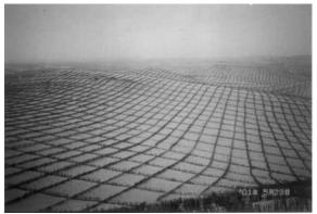
Dry straw in a checkerboard arrangement
