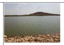
Scene of completed earthern dam, see the stone rip-rap on the upper side of the embankment
