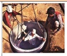
To make the construction of a hand-dug well viable, water must be available in sufficient quantities at shallow depths (6 to 25m) that will allow safe excavation and economically feasible exploitation of the water resources in the well. This will depend, of course, on local conditions, for instance it must have stable soil and a depth to the water table that does not allow pollution.
