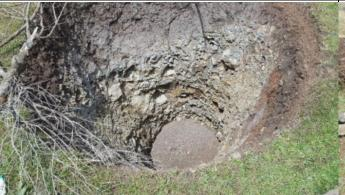
Figure 7. Percolation pit in gravely soil - cascaded in a waterway
