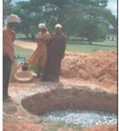
Figure 9. Excavation (left), backfilling with small stones and gravel (middle), and placement of coarse sand on top of the gravel
