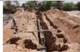
Fig 4. Subsurface dam under construction - Dire Dawa area, Ethiopia
