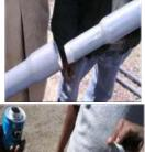
Figure 3 – Creating a socket. Heat up the end of the rising main. Insert the tool. Cool the end of the rising main with water (turn the tool around to prevent it from getting stuck). Remove the tool from the rising pipe. The socket is created.
