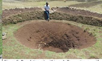
Figure 8. Percolation pit within a shallow waterway with soil embankment and stone paved spillway at the middle
