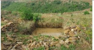
Fig. 1. Function of percolation ponds in capturing runoff and recharing of the groundwater to later be used as springs, streams and hand dug wells.
