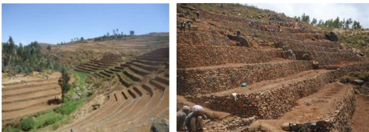
Figure 5.1 Bench Terrace On Hillside Area
