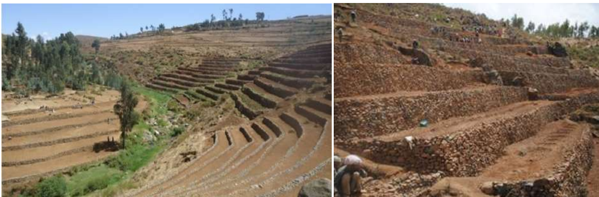
Figure 8: Bench terrace on hillside area
