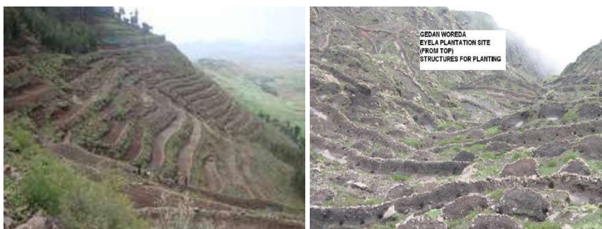
Figure 5.16 Moisture harvesting structures in steep slope areas for seedling planning purpose, photo taken from ORDA Greening Programme annual report, 2005
