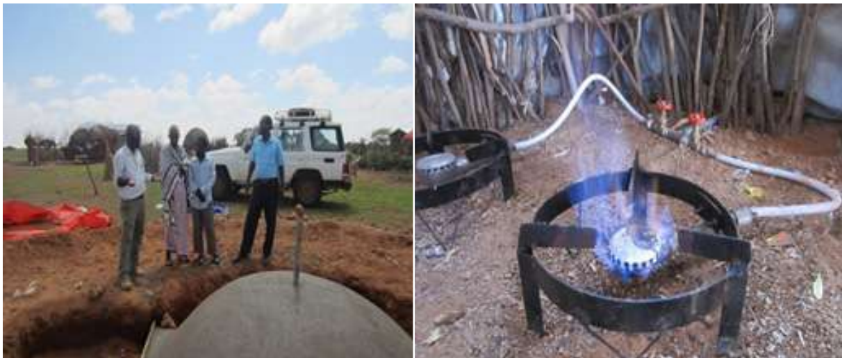
Figure 5.18 Strong flam from the biogas digester
