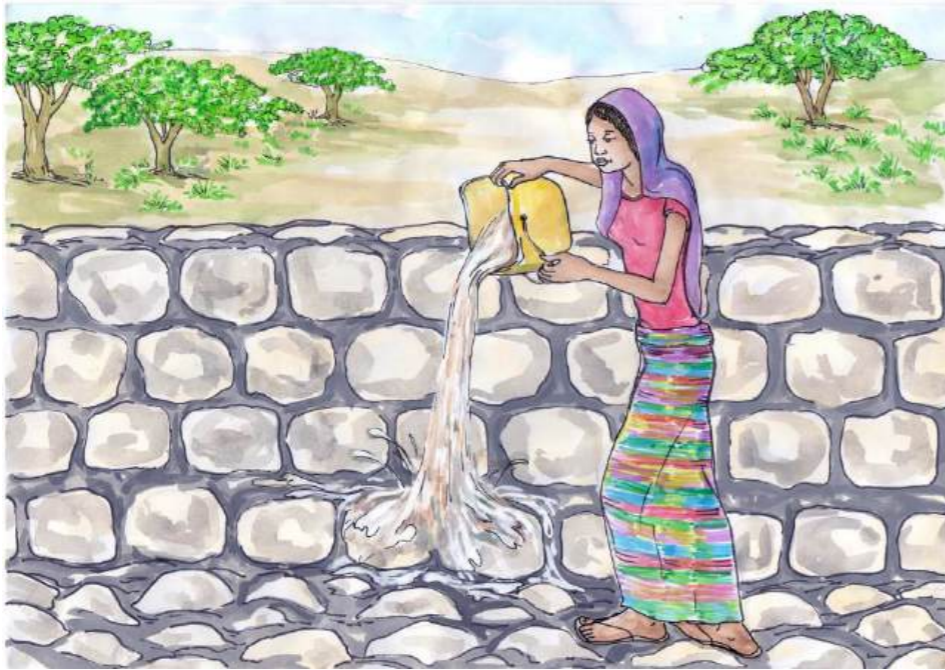
Figure 27: Watering the newly constructed WSW
