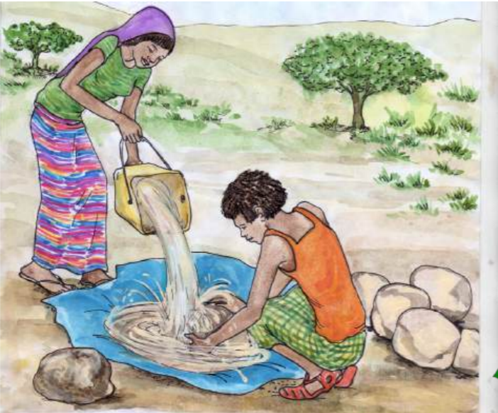
Remove dirt from stones before constructing with them.
