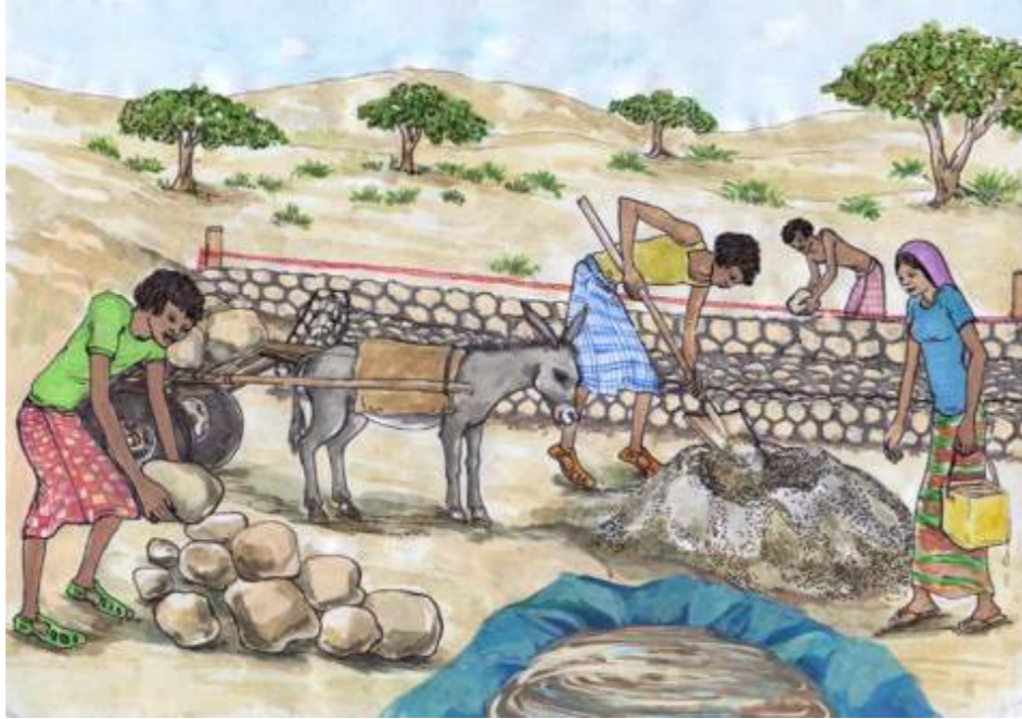
Figure 13: Construction site for a Water Spreading Weir
