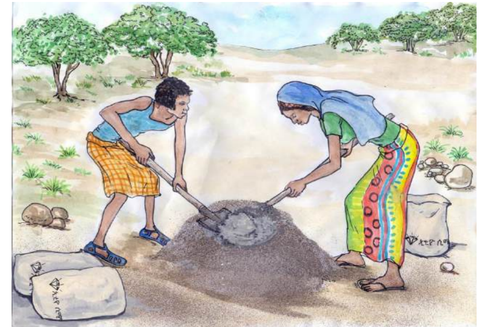
Figure 14: Mixing the mortar with sand, cement and water
