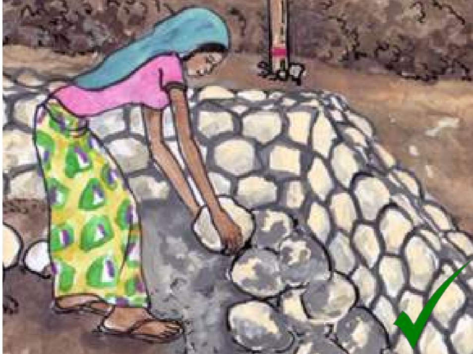
Place the stones as close as possible
