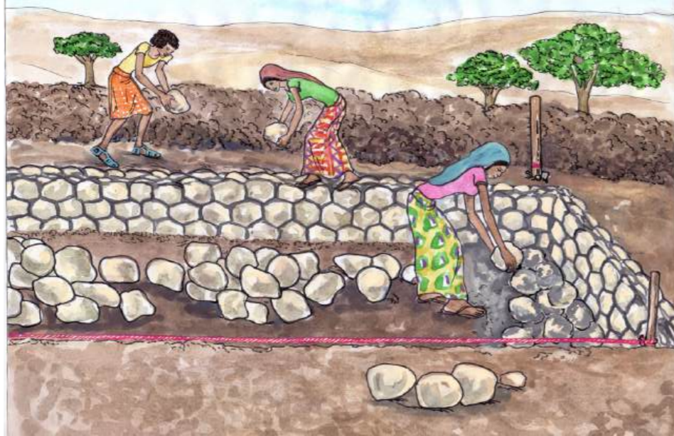
Figure 25: Under construction basin structure
