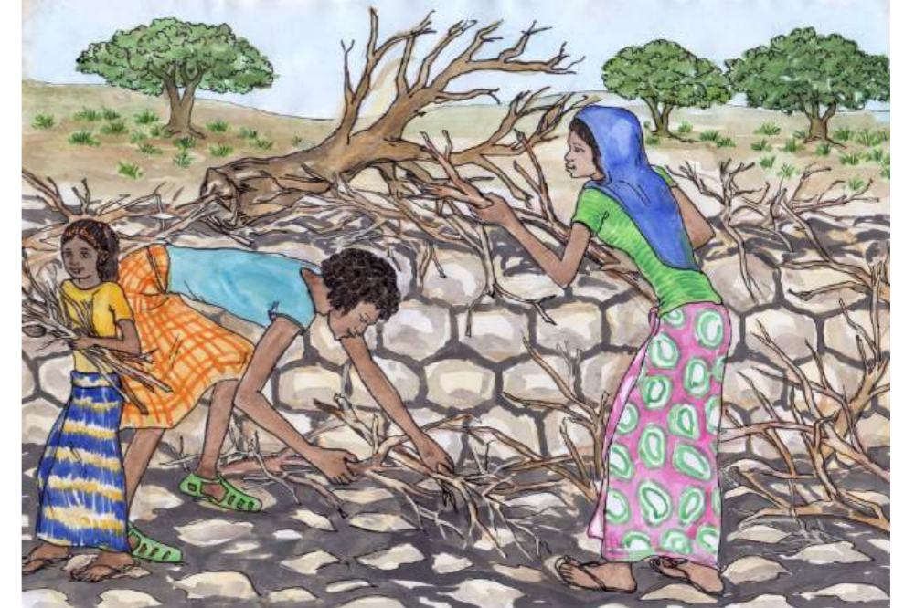
Figure 26: Covering the constructed WSW to ensure good curing
