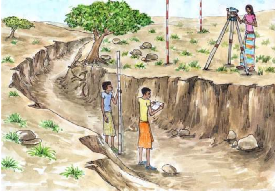
Figure 7: Setting out the WSW
