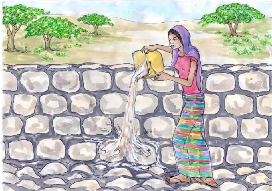
Figure 27: Watering the newly constructed WSW
