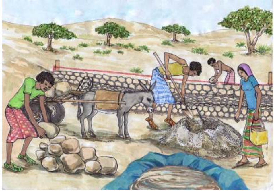
Figure 13: Construction site for a Water Spreading Weir
