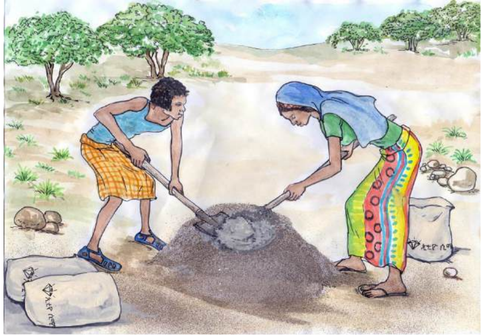
Figure 14: Mixing the mortar with sand, cement and water
