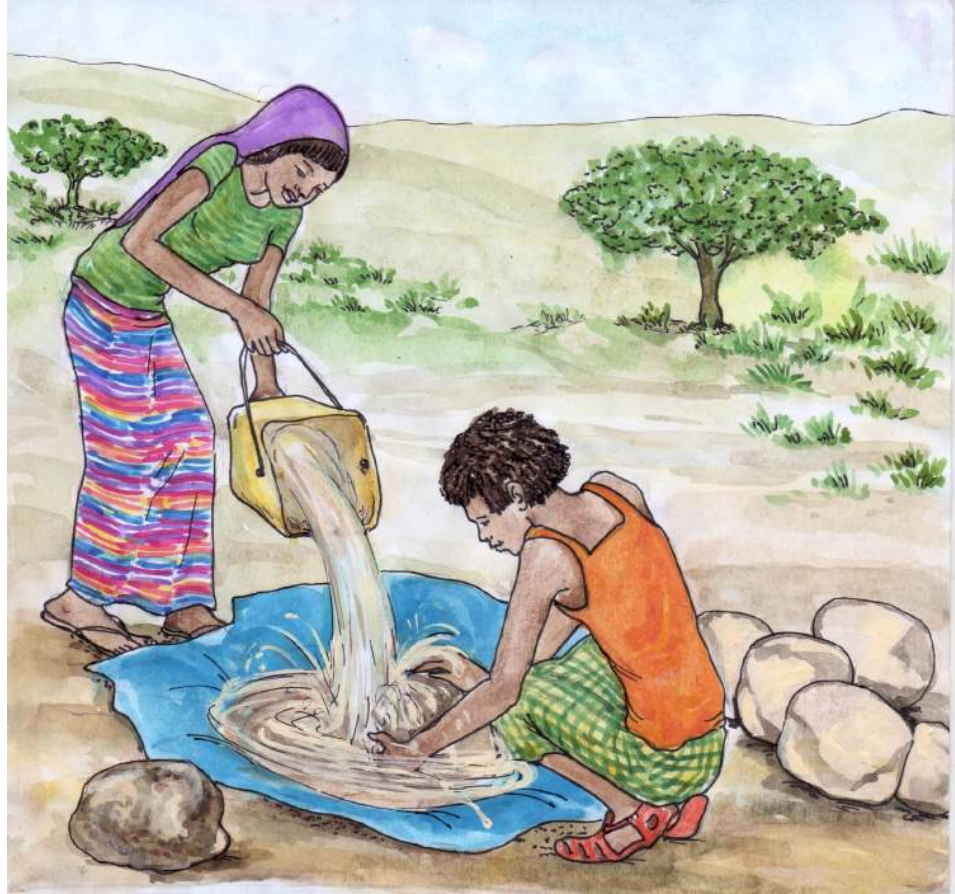
Figure 16: Washing stones before using them in the WSW
