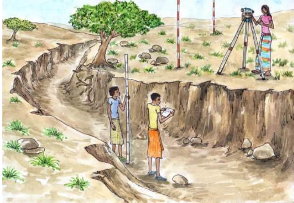
Figure 7: Setting out the WSW
