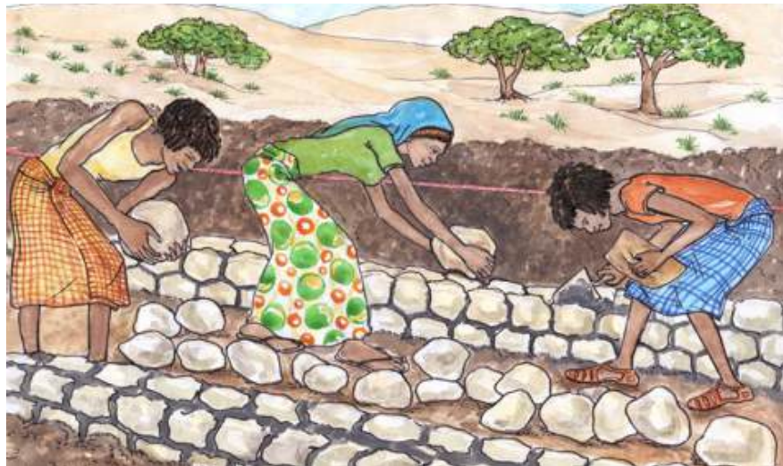
Figure 18: Constructing the main wall
