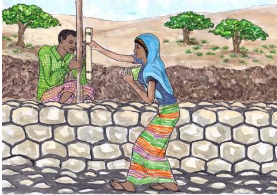
Figure 28: Checking the levelling of the WSW as part of quality control
