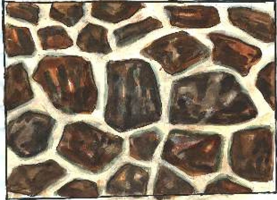
Figure 20: Detail of constructed wall showing the stone shape
