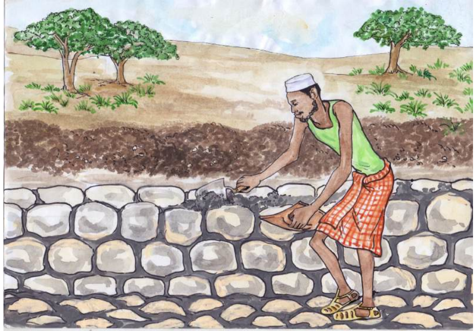
Figure 21: finishing the wall
