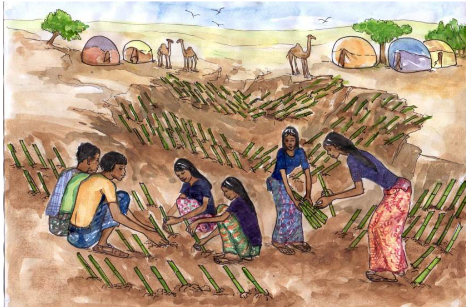
Figure 14: Inserting the cuttings in the flood of the gully, to start the biological check dam
