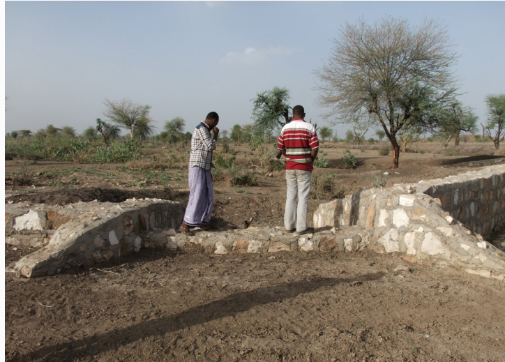
Picture 3: Transect walk to assess the state of the structures.
