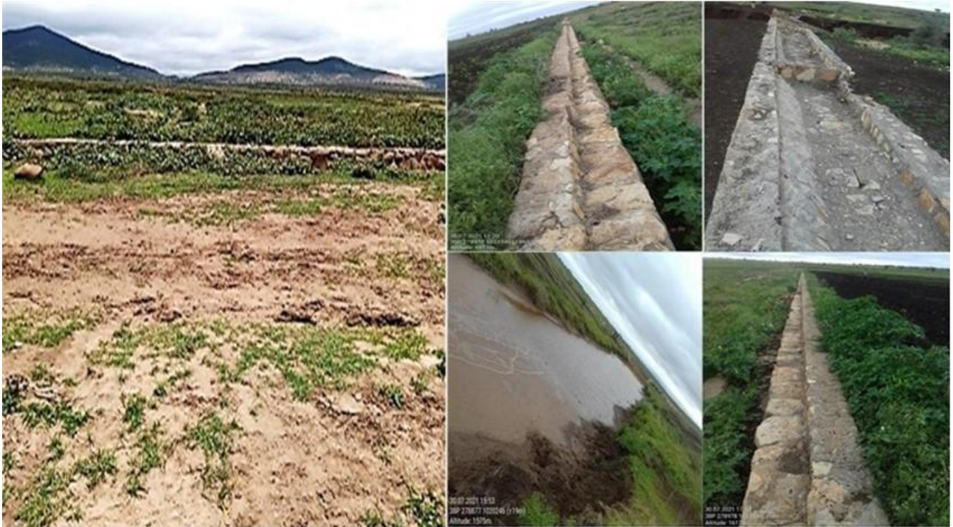
Picture 3: Photo-water spreading Weir technology in Gubka and Harre Dry valley project Sites
