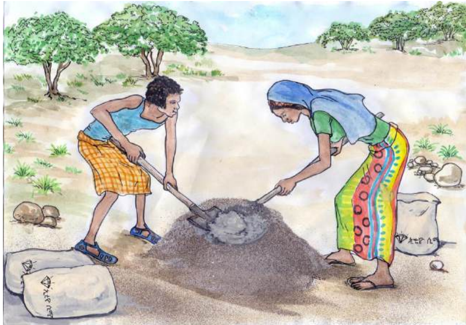
Illustration 23: Sand and cement are mixed.
