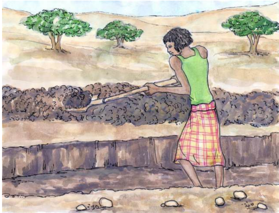
Illustration 41: Place excavated soil on the upper side of the weir, at the end of construction soil is filled back right up to the finished walls.
