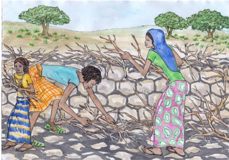
Illustration 52: good rains have flooded the land and brought sedimentation. Removing branches and stems of trees is an easy maintenance work to be done by the maintenance team itself or a small community group.
