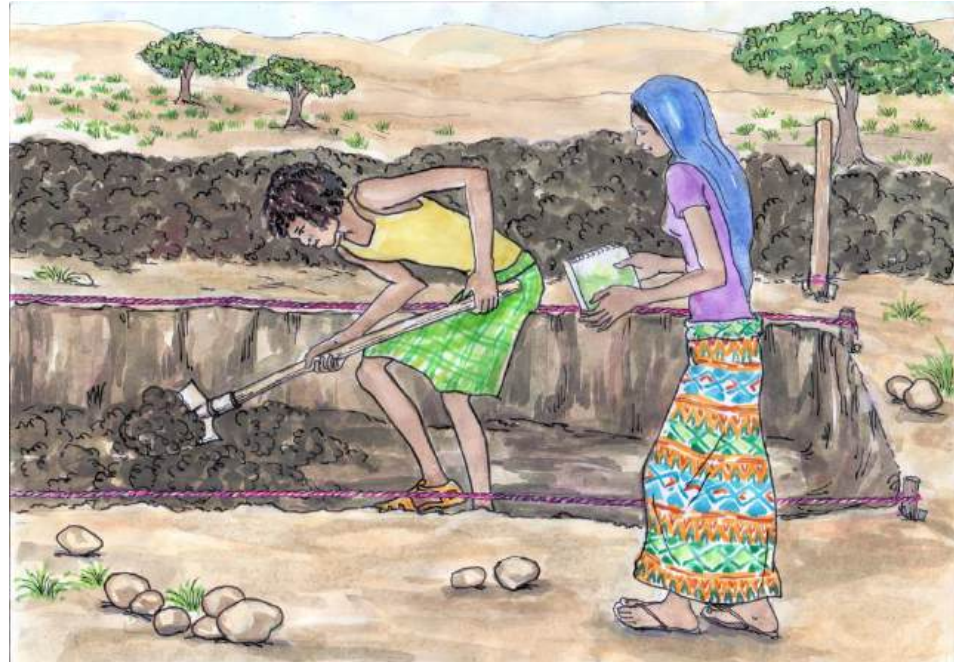
Illustration 27: Excavation of the main spill over basin in the riverbed itself. The DA is supporting the supervision of the work.
