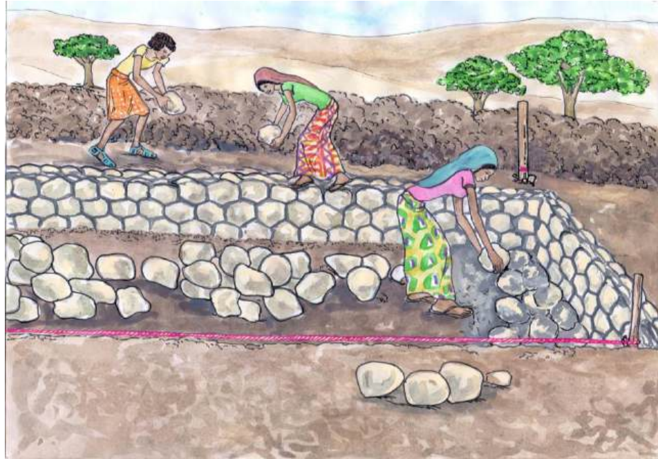
Illustration 24: Preparing the foundation of the basins of the wings.
