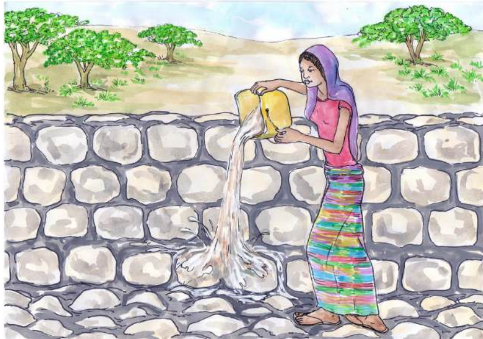
Illustration 28: watering of completed walls is extremely important.
