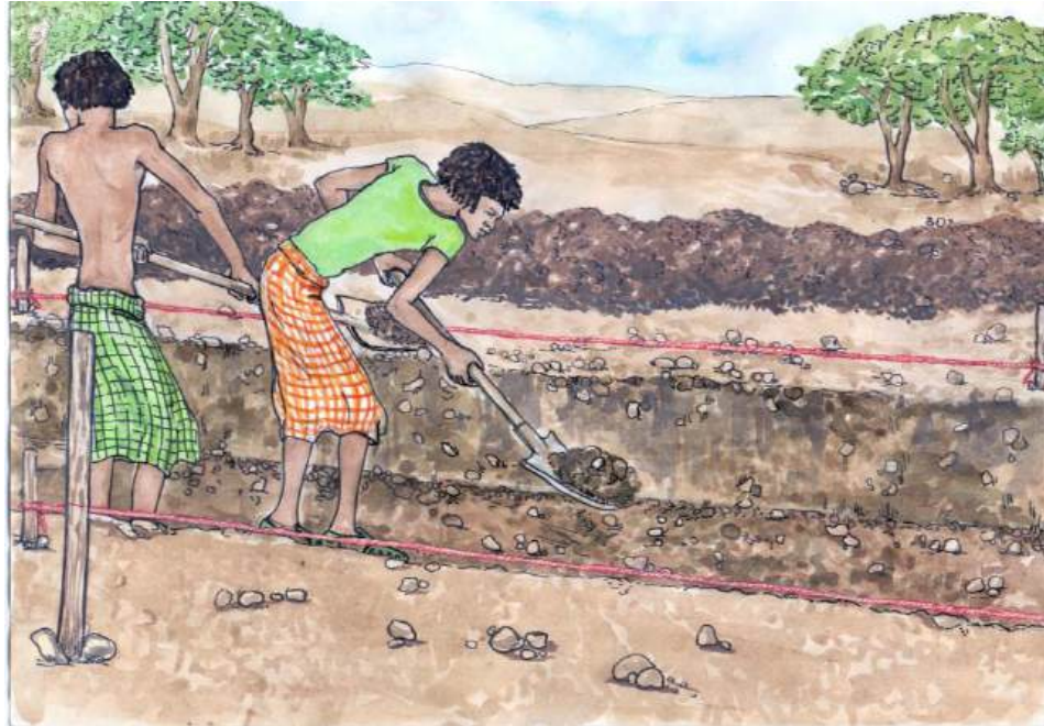
Illustration 21: the excavation for the wing to one side of the center of the weirs about 150 meters long, it ends in a shallow wall and will be combined with a drystone measure to control erosion of a smaller gully on the outer end
