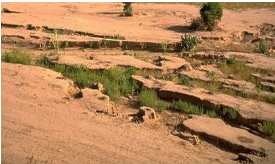
Figure 9: drainage effect by gully erosion
