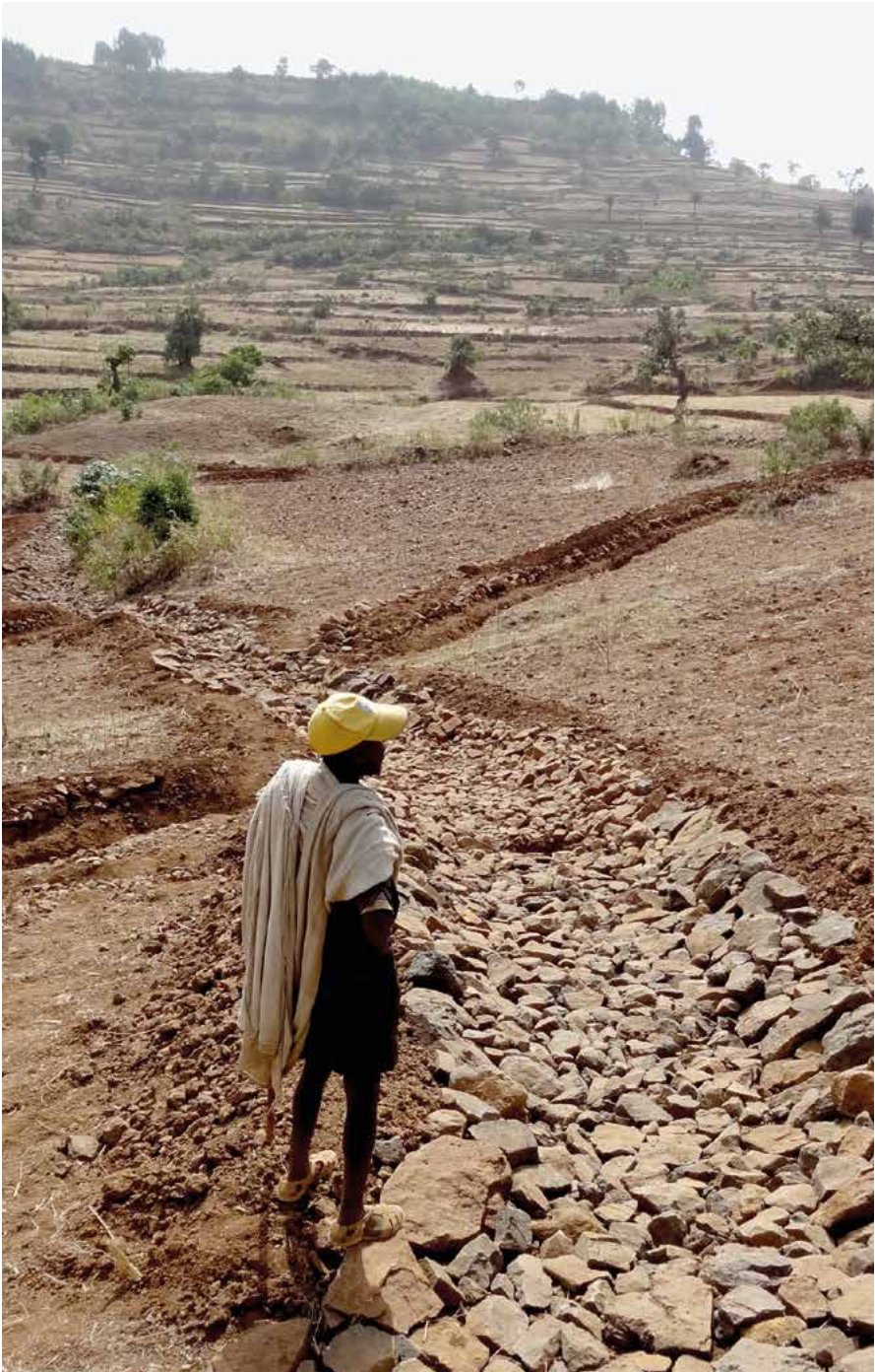
Stone-paved Cutoff Drain in Abagerima area, South Gondar (2013).
