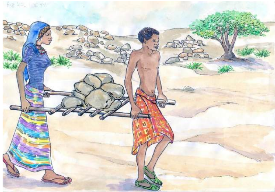
Illustration 25: Women and men can carry stones by simple traditional means, if stones are found nearby the construction site and stones are not too heavy.
