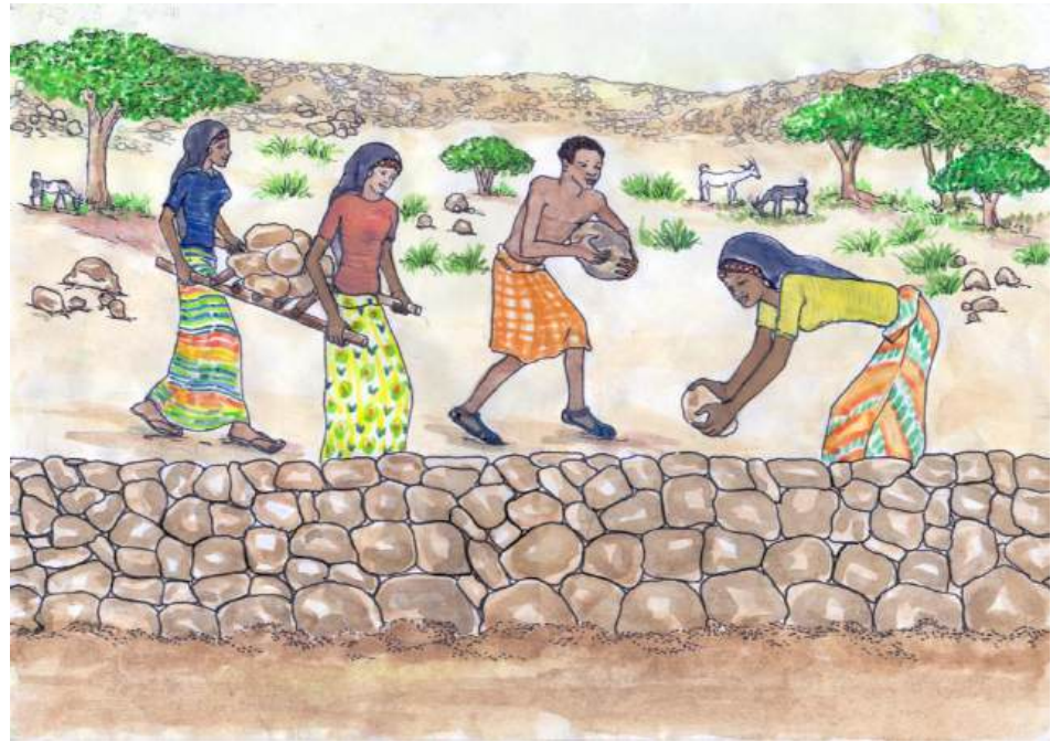
Illustration 19: Drystone structure, almost finalized. Women and men bring big flat stones to cover the small stones.
