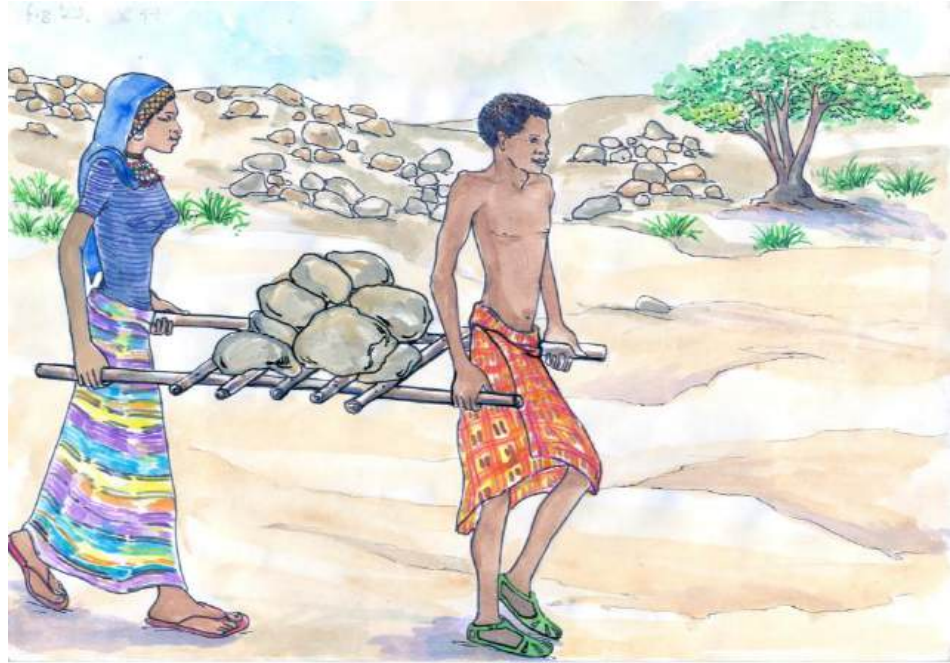
Illustration 10: If big stones are available in less than 100m distance, donkey carts are not needed for transportation
