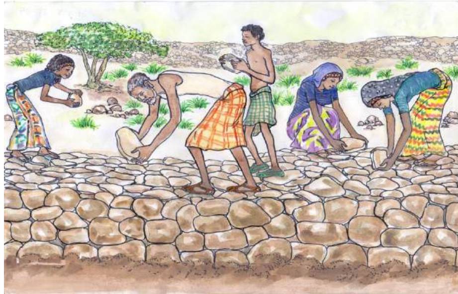
Illustration 27: community member covers the dry-stone structure with flat stones
