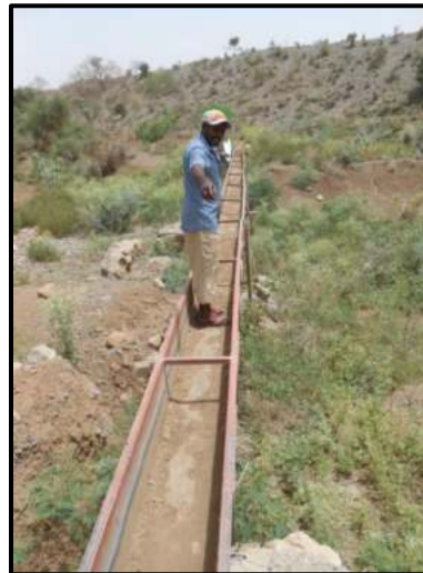
Irrigation Canal, Chifra Woreda
