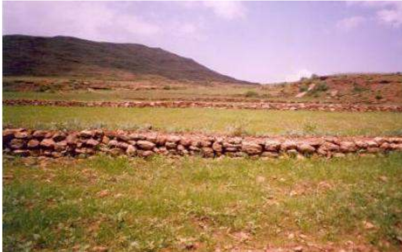
Photo 6: Double faced stone/soil bund
