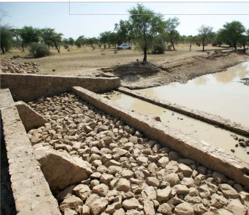
Water-spreading weir © GIZ / Klaus Wohlmann
