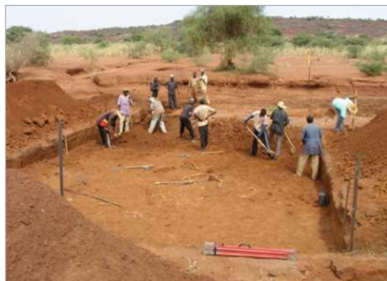
Figure 7: Training site for local craftsmen. Source: Lütjen
